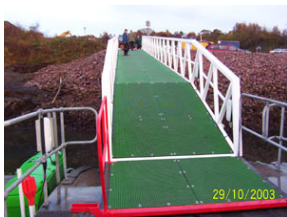
Preventing trip hazards in the wet
