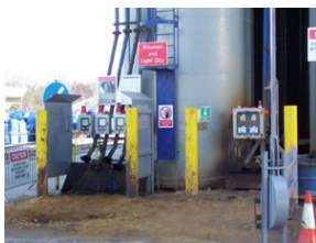
Tanker gasket failures
