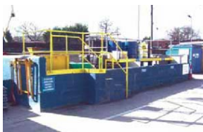
Bunded area for storage of liquids and oils
