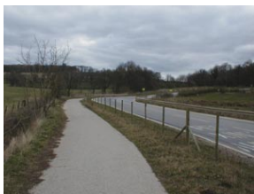
Traffic management upgrades
