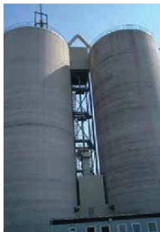
Sheltered staircase to silo roofs
