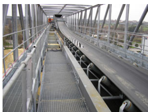
Safer access for maintenance
