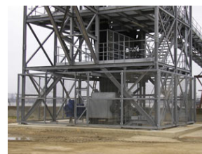
Safer access for maintenance
