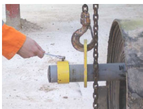
Fitting of conveyor belting
