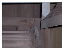
Bracket with rivet still in place
