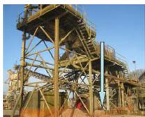
The arrow shows how the washer drum fell approximately 6-8m
