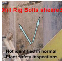
Drill rig bolts sheared
