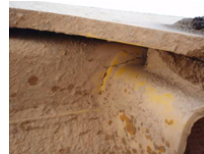
Cracks on the Tipper Body
