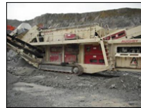
Guarded section of plant
