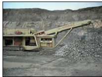
Unguarded section of plant
