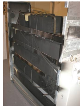
Power Supply Unit
