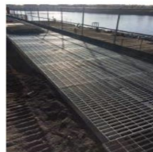
Grating secured - note overlap
