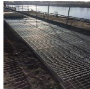
Grating secured - note overlap
