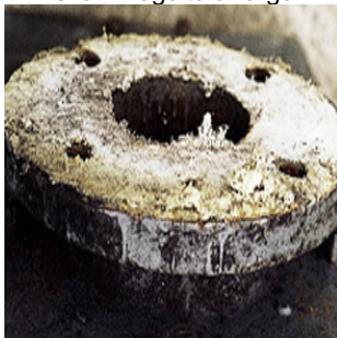
Example of an Asbestos Gasket
