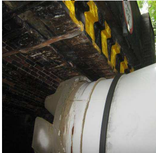
Wedged under Low Bridge
