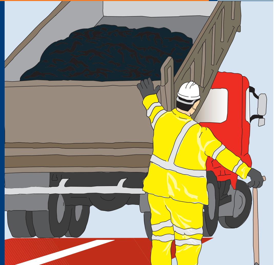
**Hand Lay** is the manual process by which asphalt, which may be at a high temperature, but sometimes cold, is removed from the back of a laden tipper vehicle via the open tailgate by the use of shovels or rakes, either into a wheelbarrow/JCB bucket or directly onto the ground, prior to spreading and rolling.
