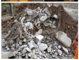
The volume of concrete that can be removed from one truck mounted drum mixer using this method.
