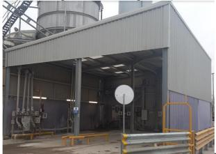
Tanker containment shed allows for the trailer to fit inside the building whilst the cab remains outside. The drivers are completely protected from the rest of the plant's operations.
