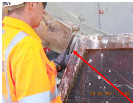
The nip point between skip and chute handle
