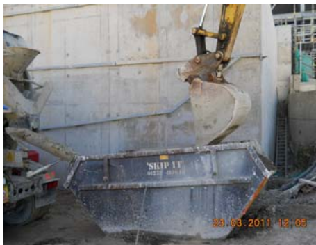
Poor delivery setup showing 360 bucket position
