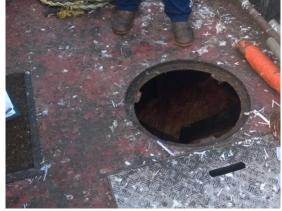
Upon lowering the first atmosphere detector into the space, it sounded a warning alarm after approximately 10 seconds. A second detector was lowered into the space by way of confirming that it was not a faulty atmosphere detector, which also alarmed providing the following results:
