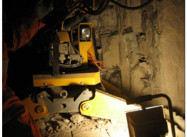
Automated wrecking by robot
