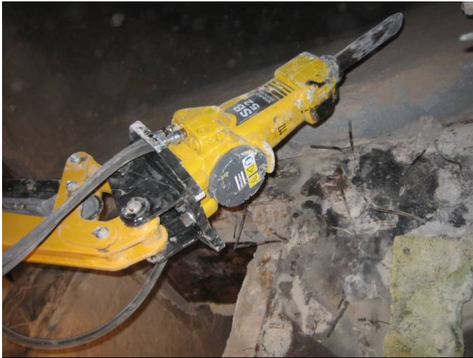
Automated wrecking by robot
