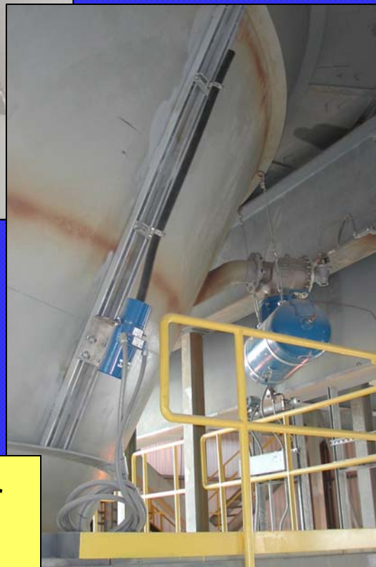
Gamma ray receiver and sensor "tail"
