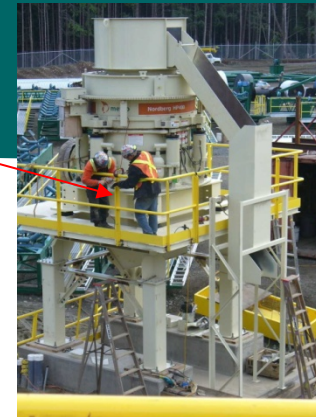
Affix Hardware for Additional Handrail Stability
