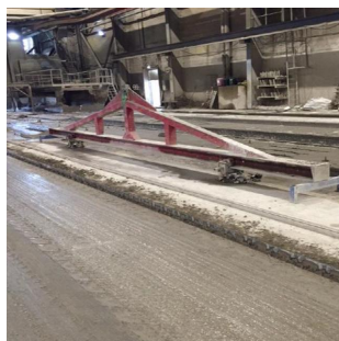
Chains on spreader beam
