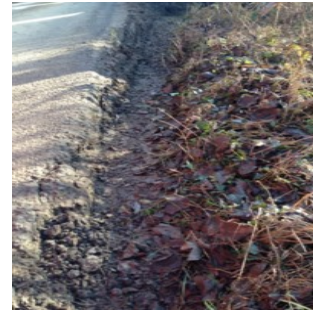
Rut to side of road
