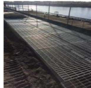
Grating secured - note overlap
