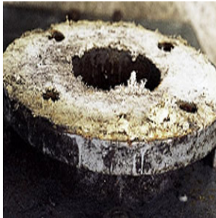
Example of an Asbestos Gasket
