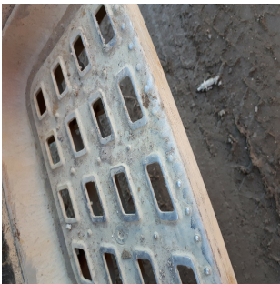
Footplate in poor condition
