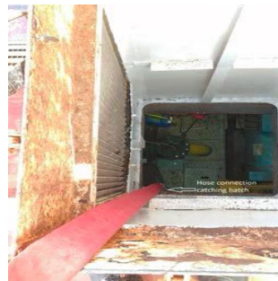
Hatch through which hose was being recovered
