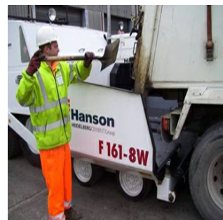
Allow spill off to flow into the paver hopper
