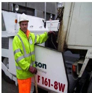
Reverse the tipper on to the paver with banks-man assistance
