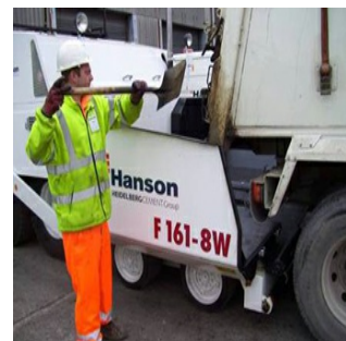
Allow spill off to flow into the paver
