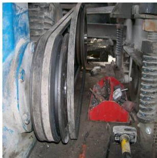
Drive belt that was being worked on
