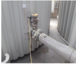
Actuator valve; with no physical way of knowing if isolated effectively
