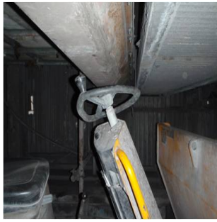
Dumper Close Up
