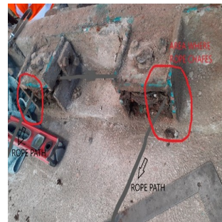
Where the wire rope was rubbing
