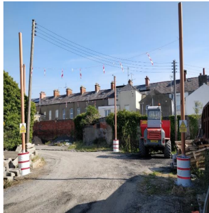
Goal posts, signage and bunting added at the site
