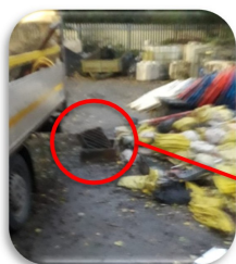
Gully left along vehicle by sandbag area
