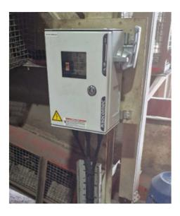
An asphalt plant engineer discovered whilst 'trying out' his isolation, that it was possible to remove his locked padlock from the isolator by depressing the handle past its 'OFF' position.
