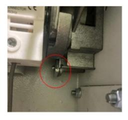
As part of the company's continual drive to reduce risk, it has recently been introducing Socomec Safety enclosure isolators into the business. These isolators are a strong robust method of isolation offering better integrity and functionality than traditional alternatives. However, this incident has highlighted that, due to this manufacturing issue, there may be flaws in some models.
