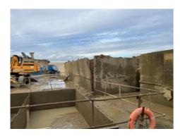
The images below show the concrete wall structural collapse and damage to edge protection to silt bays May 2024
