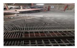
The picture below shows the opening that the employee fell through when the grid became dislodged due to previous overfill of the hopper.
