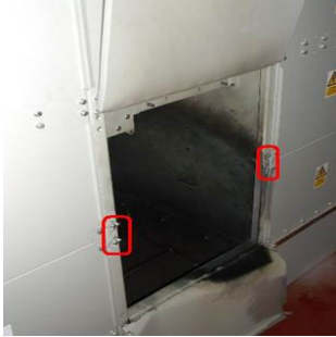
Retaining Nuts & Square Washers
