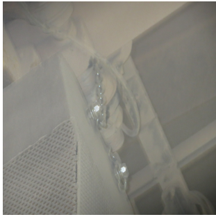
Safety chain and new box fitted.
