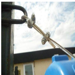
500kg plastic coated safety wire not to be used
