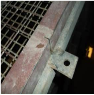
Guarding Being Cut
