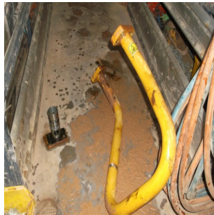
Metal Pipe Removed
