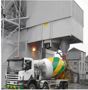
drive through loading point
