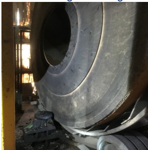
Before - shows access
