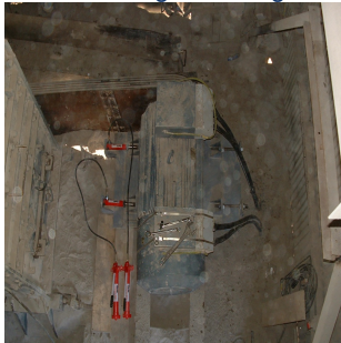
Primary crusher blow bars vibrator
