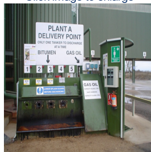
Bitumen delivery point
